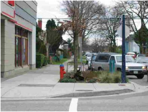
Side street with new bulges, landscaping
