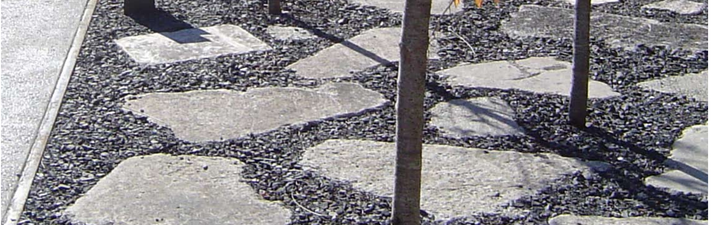
fragments of recycled concrete paving, set in gravel
