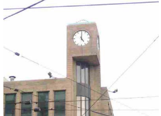
Clock at major intersection
