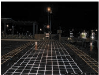
Example of Duratherm Crosswalk in Victoria, BC -low cost, plenty of designs available
